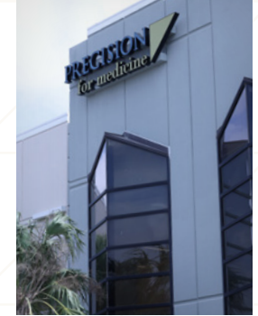
Precision's new Houston laboratory facility featuring energy efficient rooftop HVAC system LED lighting and building automation system for air and lighting.
